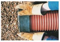
**1** Install bushes onto the square cut end of the plastic pipe.
