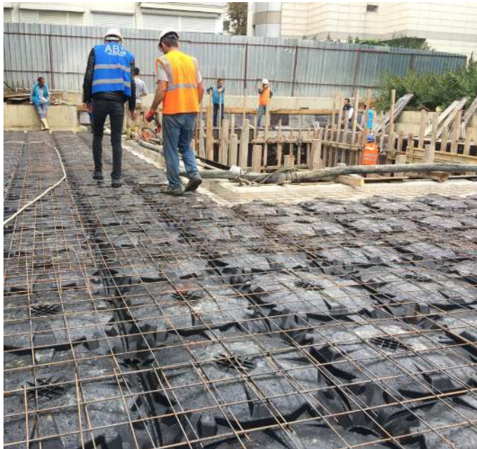
Fixed-Height Disposable Formworks For Lightweight Fillings (5,10,15cm)
